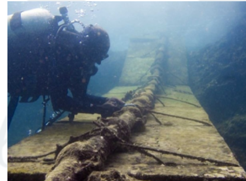
Underwater Internet cable repair
